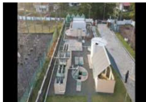
1 MLD CSTP at Padanappalam, Kannur
